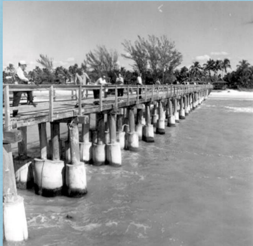
Old concrete encased pilings
