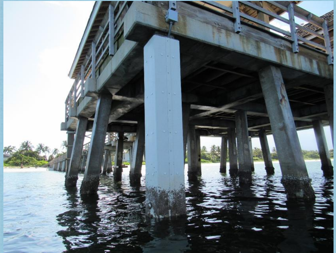
New piles encased in modern pile jackets
